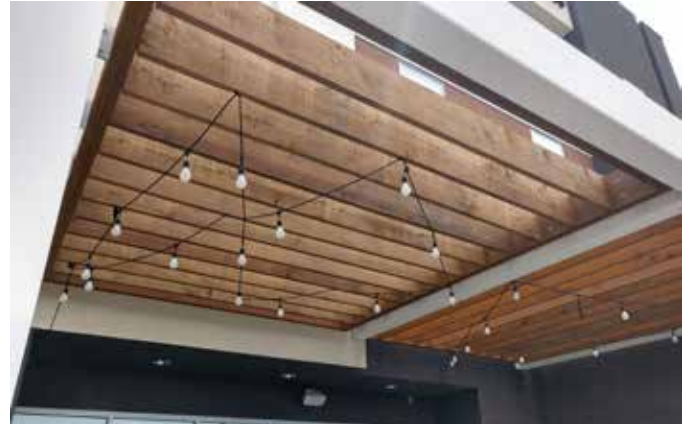
Exterior Fire-X® is often used in weather-exposed applications like this hotel pergola in Denver, CO.
