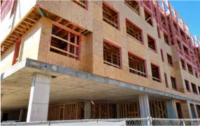
Type III with Type I podium: Pyro-Guard® used both above and below the podium. Charleston, SC.
