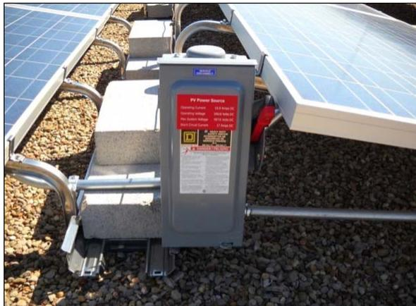
DC Disconnect Switches are usually located on roof tops for larger commercial/ industrial systems or may be on the side of a building near ground level.
