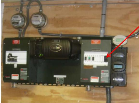
**Battery Disconnect Breaker:** The largest breaker on a battery system's power panel (which is by the inverter).
