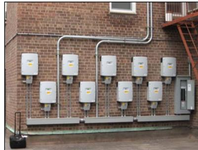
\*\*\* Review 690.31 (E) 690.14(C)(1) Exception: Installations that comply with 690.31(E) shall be permitted to have the disconnecting means located remote from the point of entry of the system conductors. 690.31(E) requires dc conductors to be run in metal raceway. This exception is very commonly used.
